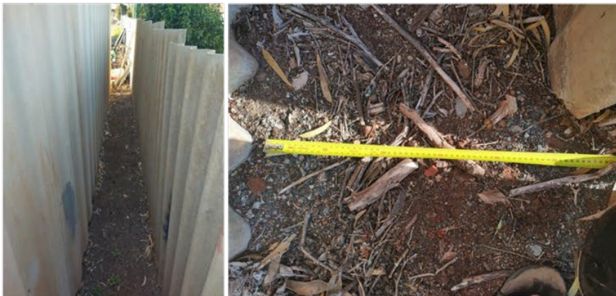
PHOTOS Current setback C (41 New Clayton Street boundary) - SIDE BOUNDARY
