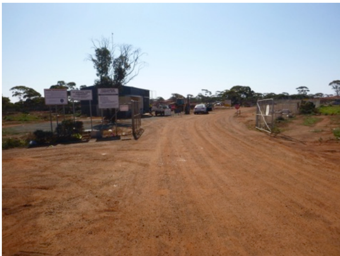
Coolgardie WMF Site Entrance
