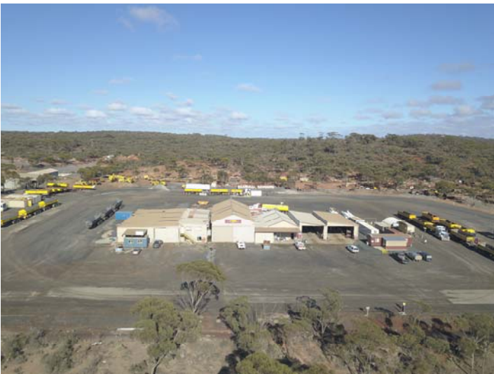
Photo of Site looking west
