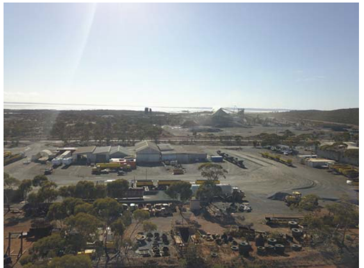
Photo of Site looking east
